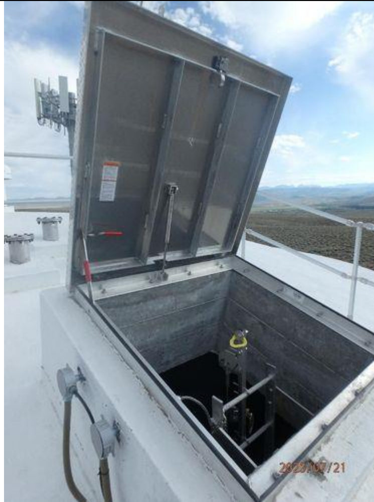
Photo # ST01-15 : Storage Tank (550k-Gal) - Hatch Gasket
