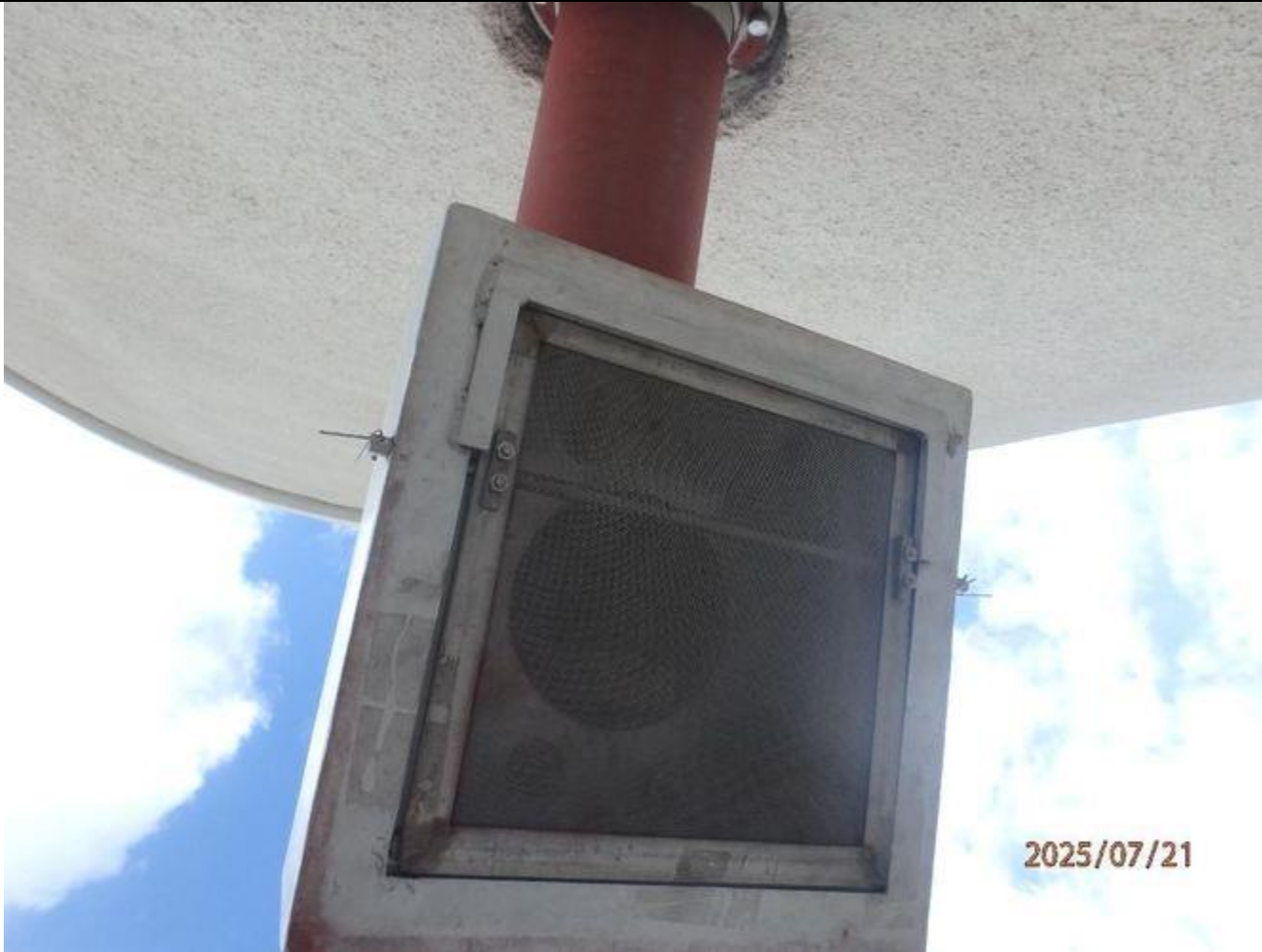
Photo # ST01-5 : Storage Tank (550k-Gal) - Overflow Screen
